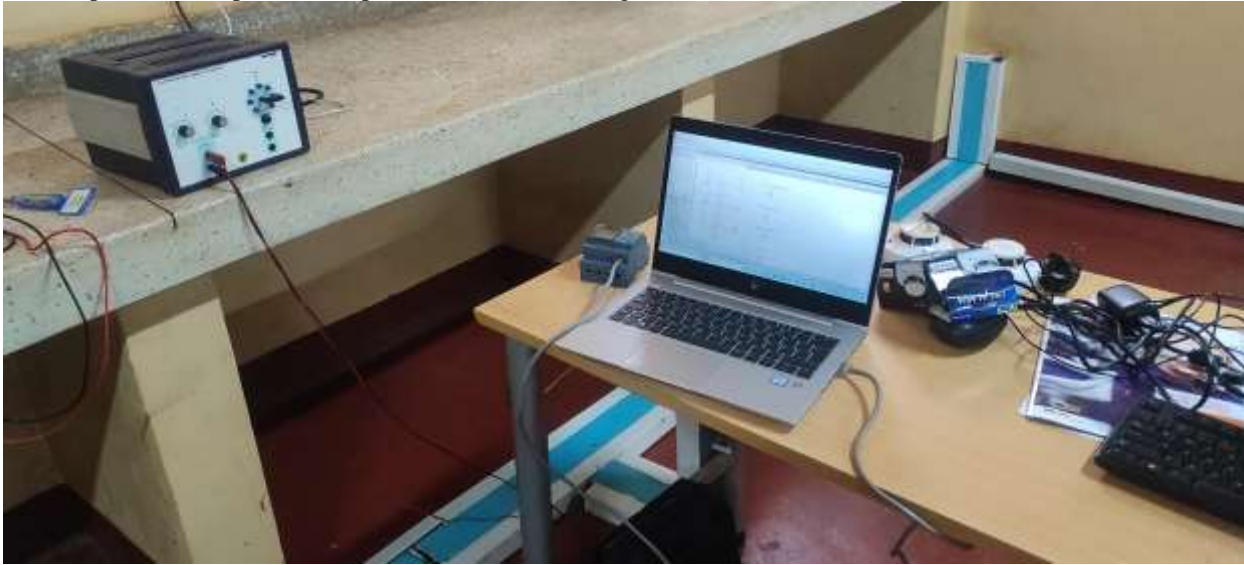
Fig. 8: Uploading the program from PC to the PLC
